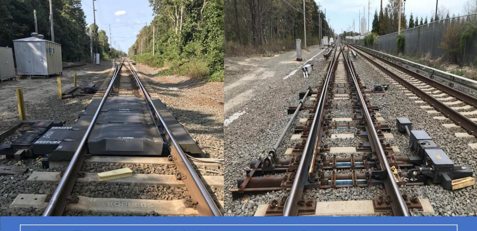
Installing new track infrastructure to harden our assets, such as snow switch covers and new switch rods and insultations.
