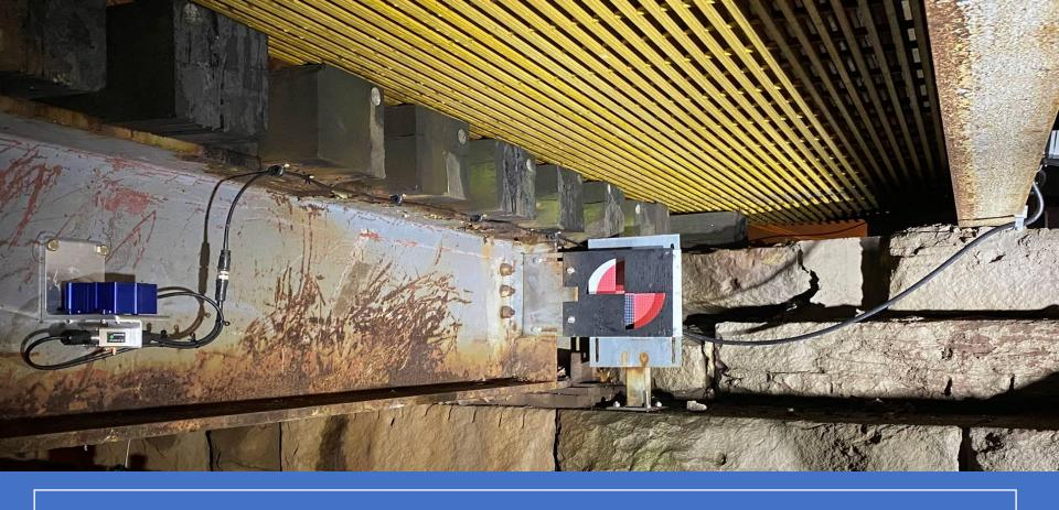
Installing bridge strike sensors and cameras on 6 different low grade bridge crossings.
